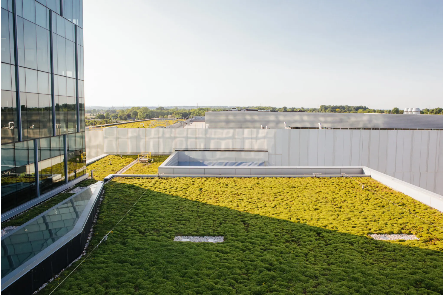
A green roof at the Air Products headquarters. Michelle Gustafson for The New York Times
